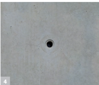
4 High quality concrete surface results with the ECOPLUS form lining
